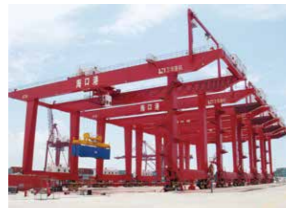
海口港轨道式集装箱门式起重机 Rail Mounted Container Gantry Crane at Haikou Port
